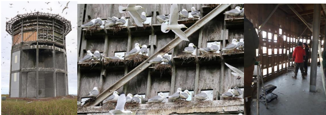
Figure 7.4: Kittiwake colony on Middleton Island, Alaska. A converted radar tower fitted with removable panels enables easy access to nest sites for supplemental feeding and monitoring. (Photos by Jon Green).
